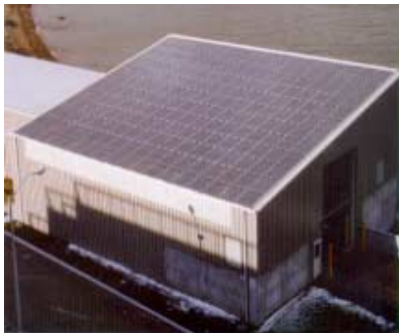
Fig. 4: Rikers Island, New Your City, 40\text{kW}_p skylight
