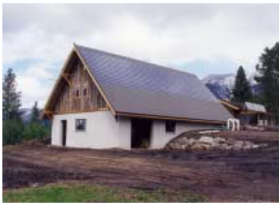
Fig. 2: Stand alone system in Montana, 12.4 kW Sunslates
